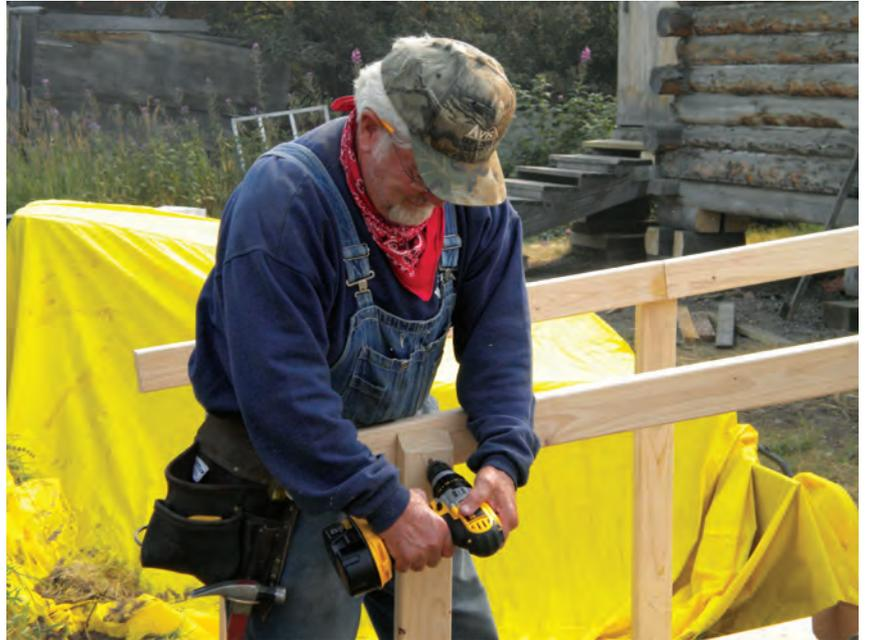
*Mennonite Disaster Service volunteer Amos Diener drills a handrail on a new handicap ramp for a home damaged by flood waters at Stevens Village, Alaska. The handicap ramp became necessary because Amos and his fellow volunteer raised the house two feet to prevent future flood damage. Photo: FEMA/Ben Brennan*
